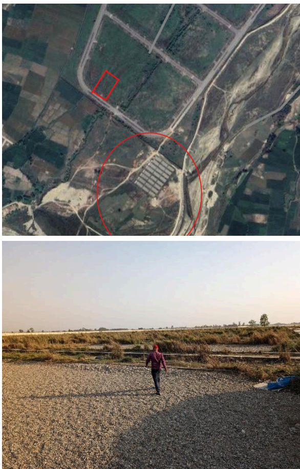
Fig: SEZ Simara wastewater treatment plant
