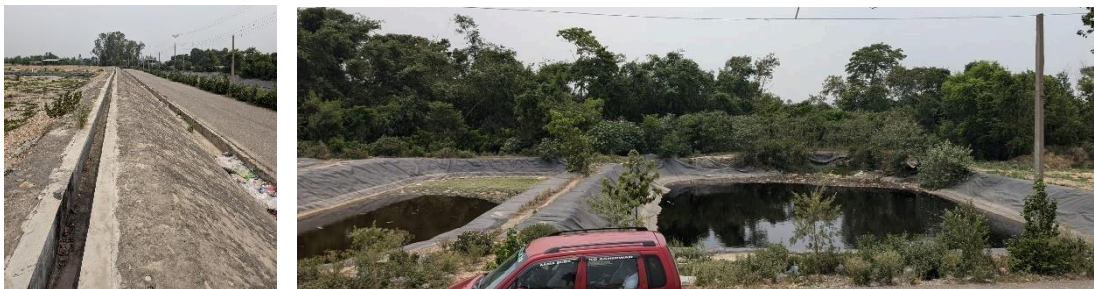
Fig: Leachate Collection Drain and Treatment Unit of Birgunj Municipality
